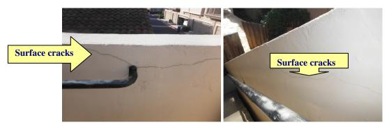
One or more sections of the rear staircase (top railing) wall were noted with surface cracks. We recommend sealing all surface cracks. Doing so will help prevent moisture intrusion within the cavity of the wall.
